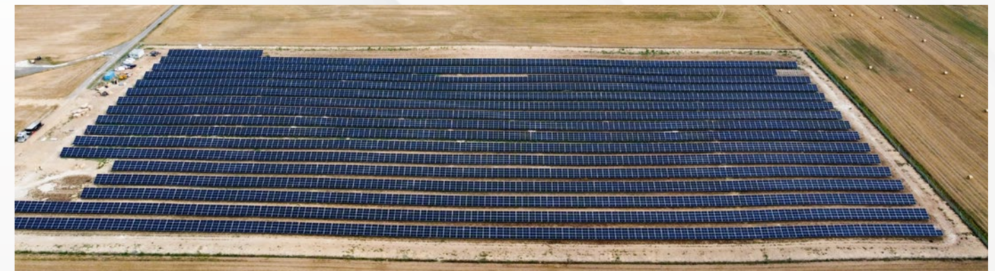
Photograph of a 5MW Prestressed Concrete installation
